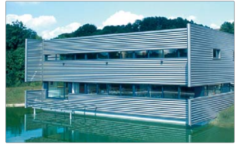
interscience R&D center and manufacturing plant Mourjou FRANCE
